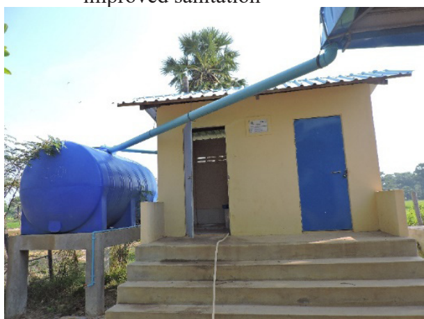
Figure 9: Flood-resilient latrine and rainwater collection/storage system for improved sanitation
