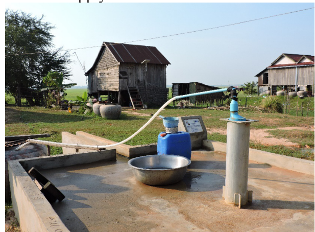
Figure 8: Water pump for year-round water supply
